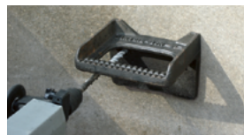
5. Drill and clean second hole. Step iron serves as plate drill jig.
