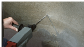
Easy installation - quick and reliable embedment: 1. Drill hole.
