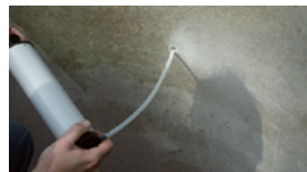
2. Clean drill hole.
