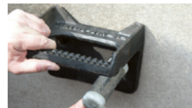
3. Place the step iron anchor through the hole in the step iron using the push-through method.
